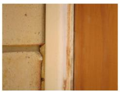
e) The pipework to the downpipe behind the wall at the front left hand corner of the house is full of sand. No undermining of the footings is occurring but it is recommended the pipework be repaired.
