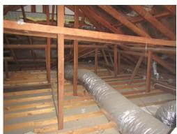
b) The roof is insulated with anticon insulation under the roof sheeting. It is recommended insulation be installed on top of the ceiling to further increase the energy efficiency of the home.
